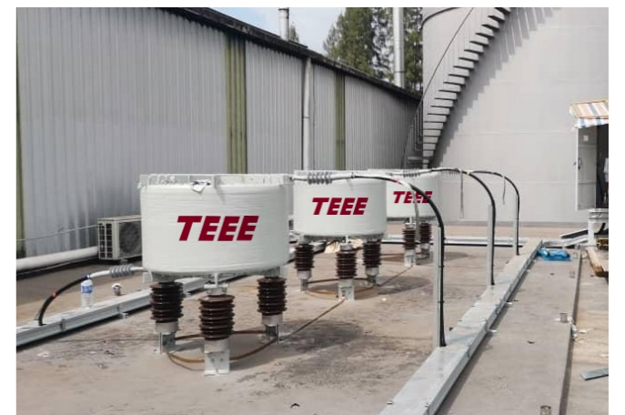
Malaysia Project 300A Current Limiting Reactor
