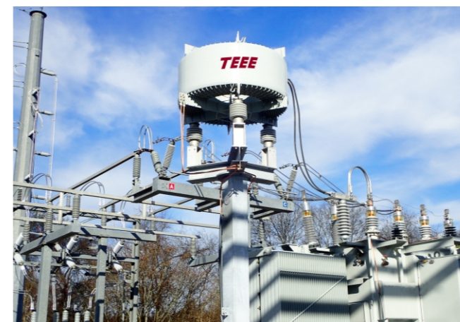
Knoxville Utilities Board Project in U.S 875A Neutral Grounding Reactor
