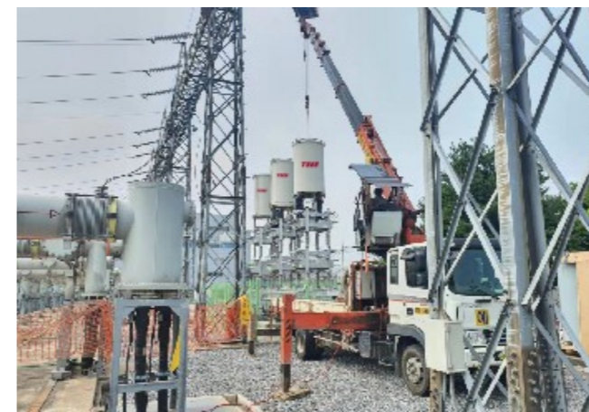
Job No.229306 KEPCO PJT in South Korea 170kV Current Limiting Reactor
