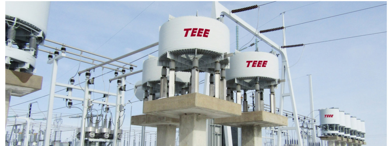
NPPD Project in the U.S. 6667kVA Shunt Reactor
