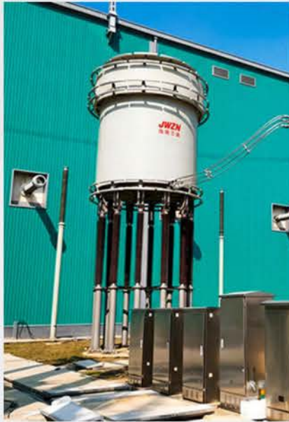
Baihetan - Jiangsu ±800 kV UHVDC project 500kV Converter Reactor-LV
