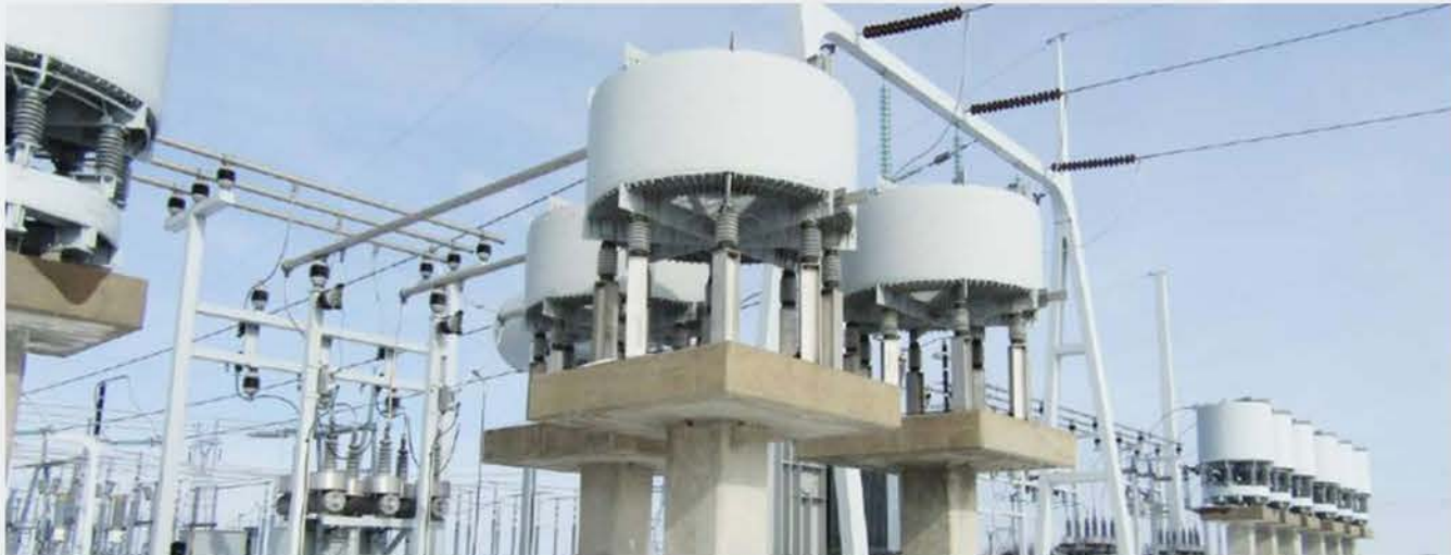
NPPD Project in the U.S. 6667kVA Shunt Reactor
